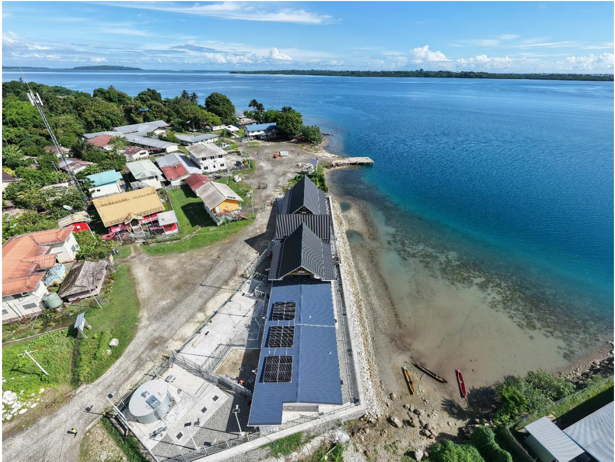
Photo 3 - The soon-to-open Buala Market is Solomon Islands' first market purpose-built to be inclusive and accessible, as well as featuring a climate resilient seawall and solar power.
